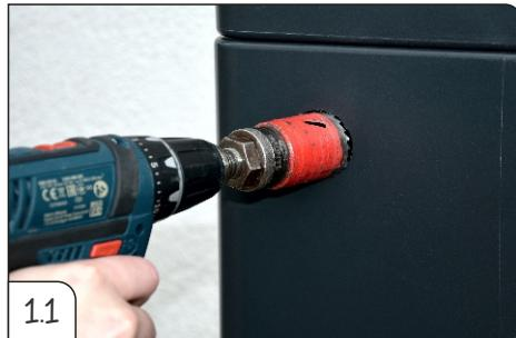
**1.2 Durchführungsgummi ① in die Bohrung einsetzen.**
